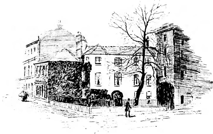
HOUSE AT THE CORNER OF CHICHESTER STREET AND CALLENDER STREET.
